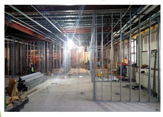
Metal stud framing for the new layout is nearing completion.
