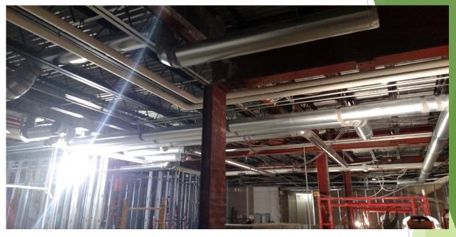
Underground plumbing for the new office bathroom has been completed and new duct work for the main office is in place.
